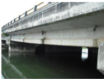
(a) Concrete girder bridge
