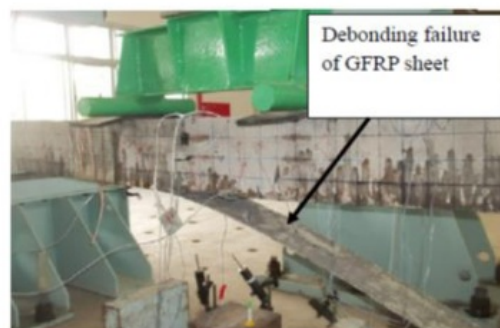
Fig.8. Debonding failure of GFRP sheet.
