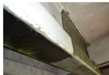
(b) Strengthened girder using GFRP sheet
